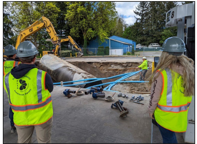
Removal of a UST (Source: PLIA)
