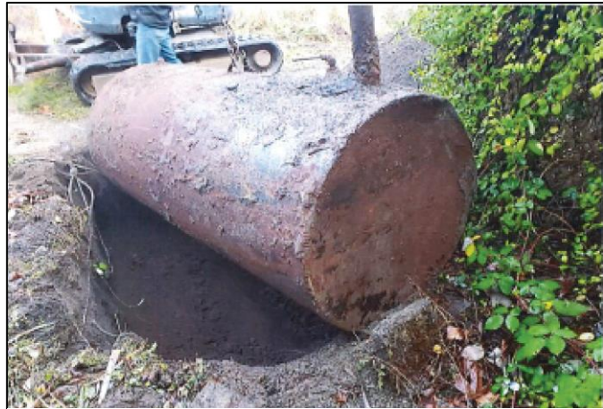
Heating Oil Tank removal (Source: Langseth Environmental Services Inc.)
