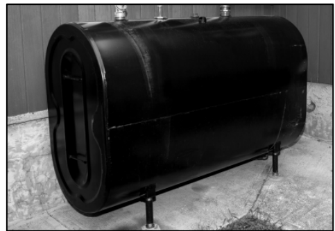
Heating Oil Tank (source: Michigan.gov).
